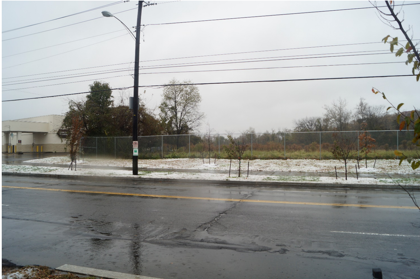
Final view of site as seen from South Capitol Street
